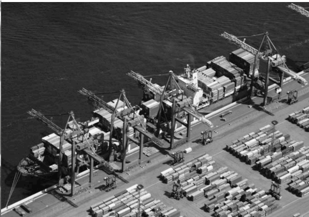
Quay crane (Meisel, 2009)
