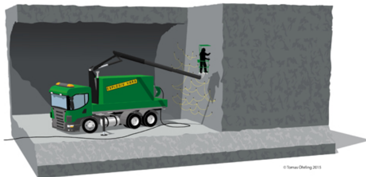
Figure 2.5: Illustration of the second activity in the Blasting Cycle - Charging . Source: Copyright 2015 by Tomas Öhrling with permission.
