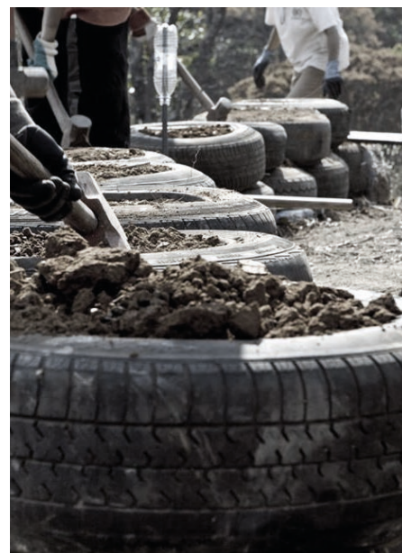
Earthship construction. Image Jenny Parkins
