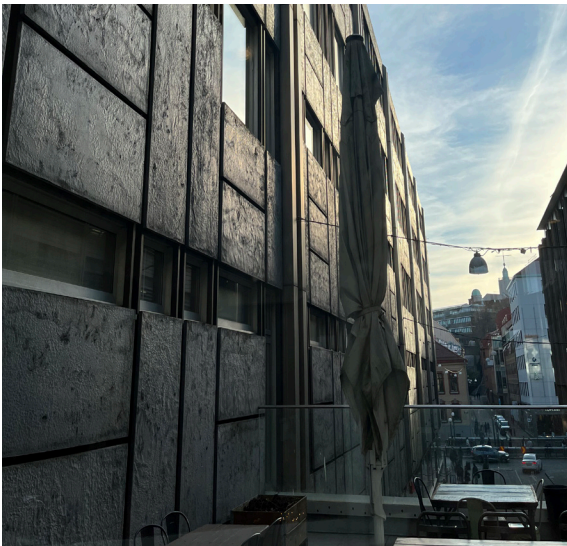
Figure 31. Photo by author. Western side, Spannmålsgränd.
