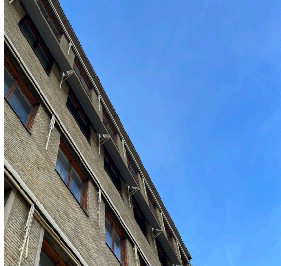
Figure 30. Photo by author. North western corner, towards Norra Hamngatan.
