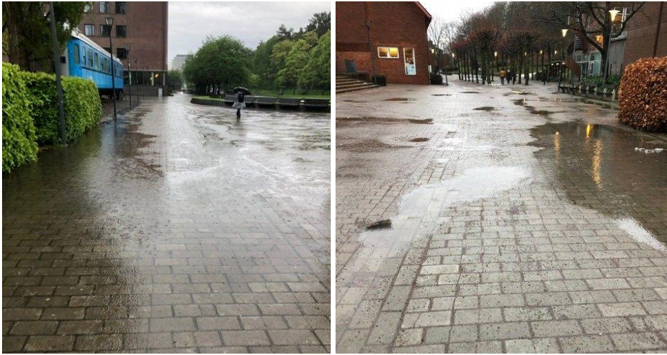
Figure 16. Passage during rain.
