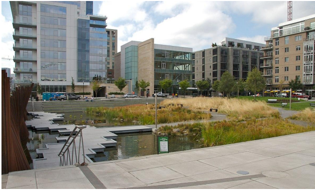
Figure 7. An example of a multifunctional stormwater solution. The image depicts Tanner Springs Park in Seattle, USA. While offering a green space and meeting space, the park also acts as a stormwater retention pond during heavy rainfall and flooding. From Tanner Springs Park [Photograph] by Cord Rodefield, 2007, Wikimedia Commons.
