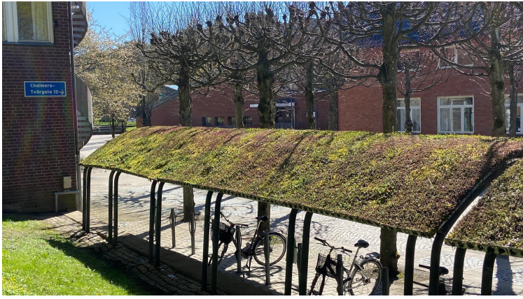
Figure 4. Example of a green roof.
