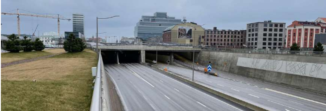
Figure 3.0.2: View of the lowering, retaining walls and entrance of the tunnel.
