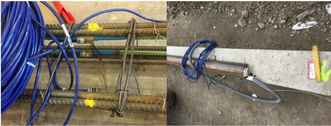
(a) Strain gauge installation.
