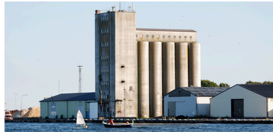
The former silo was a prominent landmark in Bergkvara, as seen here in 2008.
