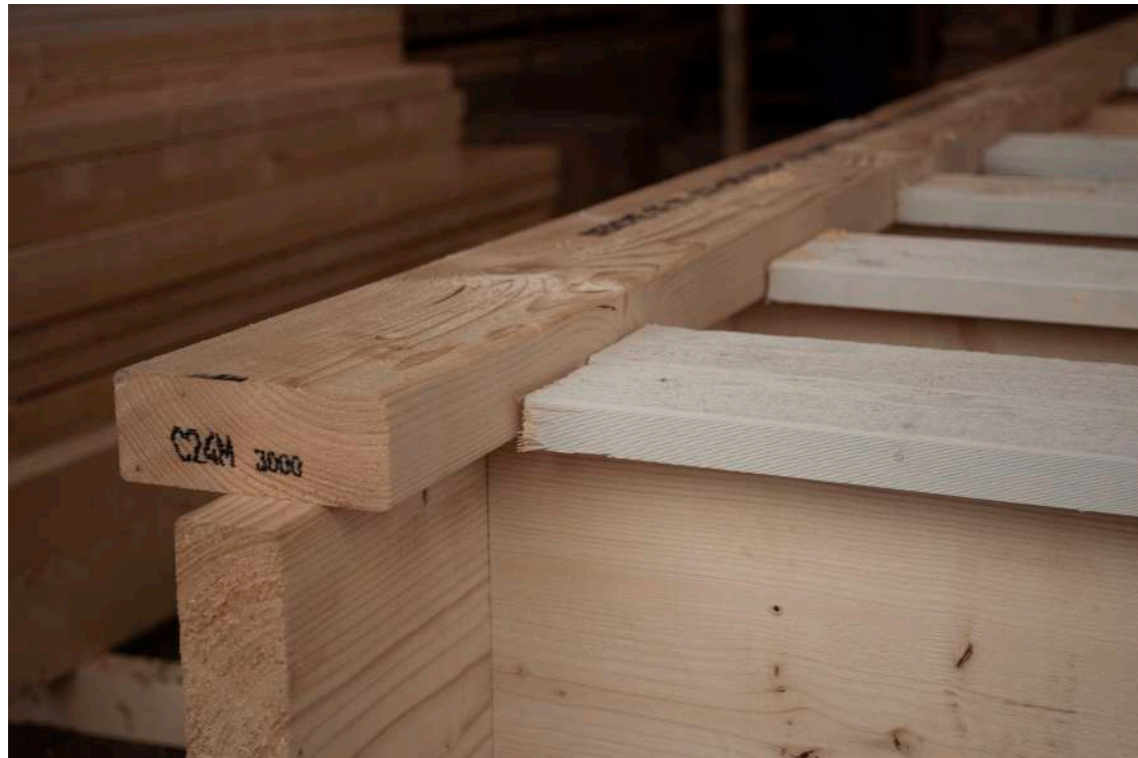
Image 25. Resued wood underneath the floor structure. March 12
