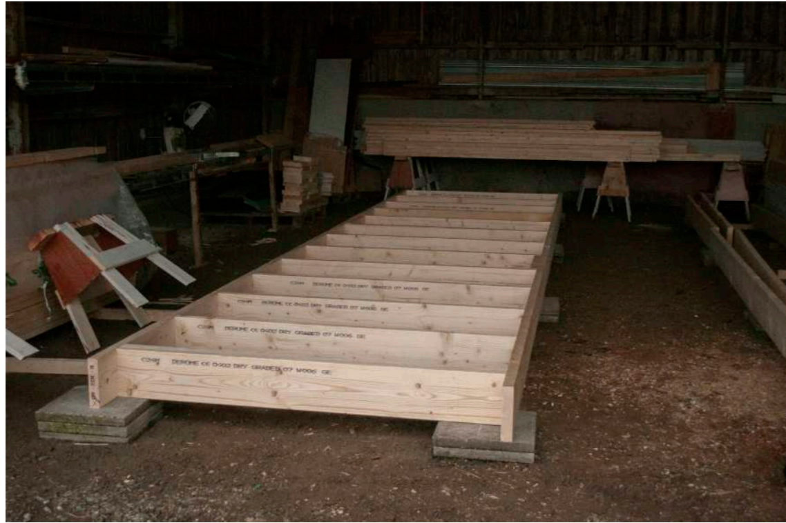
Image 24. First half of the floor structure. March 11
