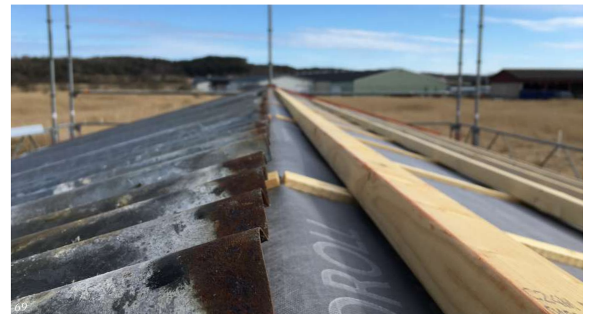
Image 65-69. Mounting of metal sheets and closing the holes. April 14
