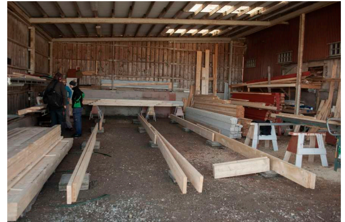
Image 23. Start of the floor structure. March 11
