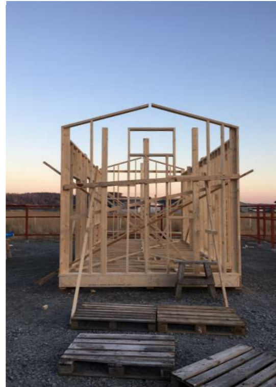
Image 44. Assembling the rest of the walls. March 26
