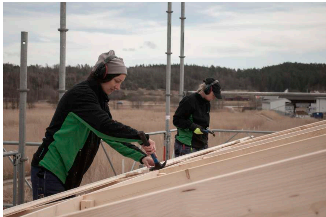
Image 52. Mounting of tongue and groove. April 1
