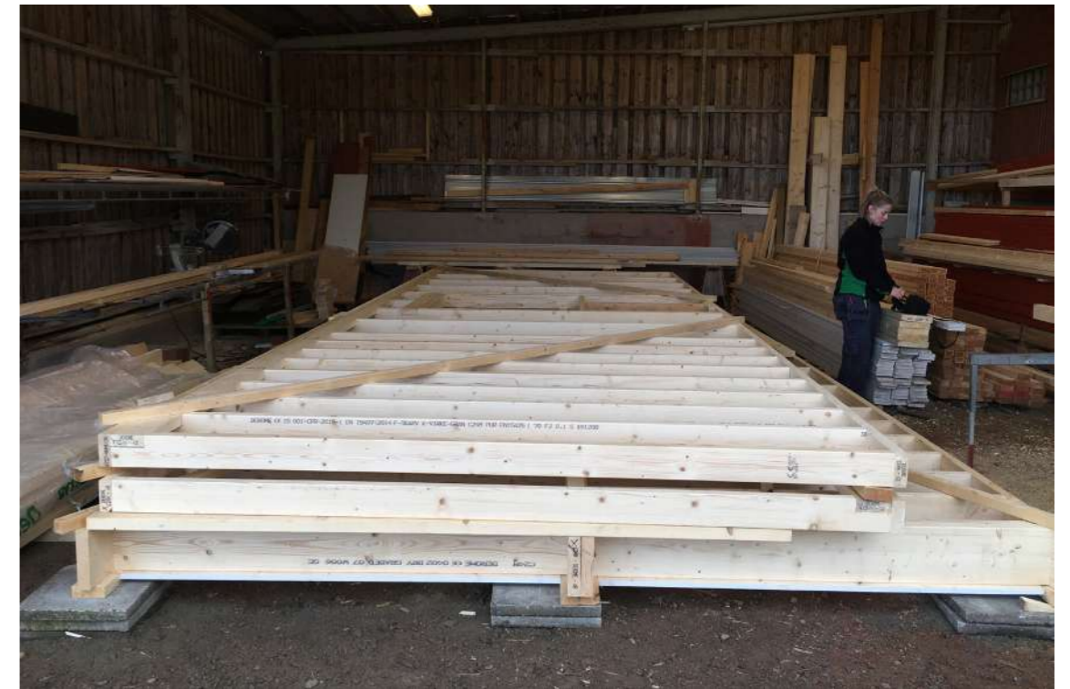
Image 30. Walls were built on top of the floor structure. March 16
