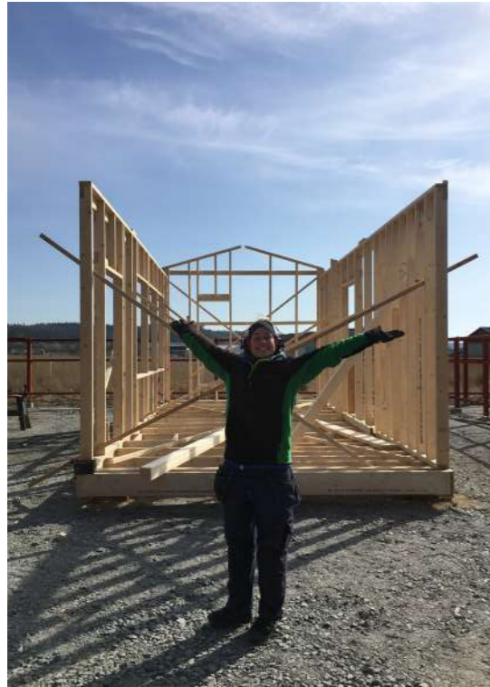
Image 43. Assembling the rest of the walls. March 25
