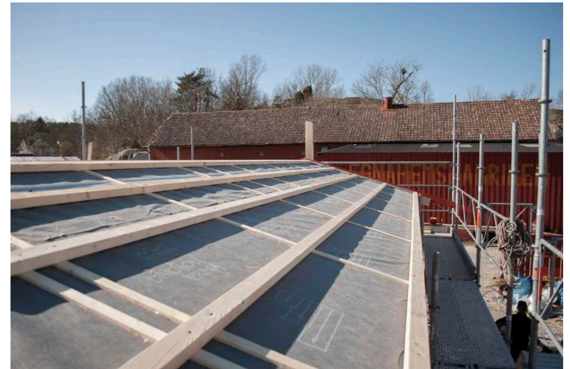
Image 56. Sarking membrane and wooden battens mounted on the roof. April 7
