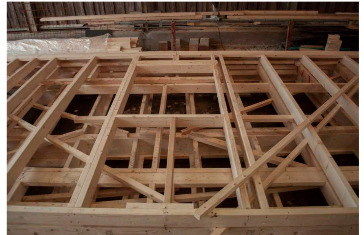
Image 29. Moving a window during construction. March 16
