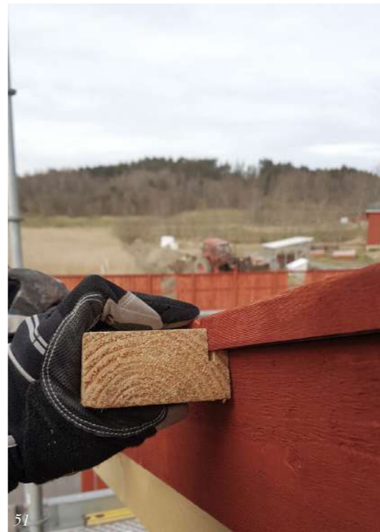
Image 50-51. Some tips and tricks from one of the carpenters. If several similar parts are to be constructed or mounted, it is easier to get it right by creating different templates to use. April 1
