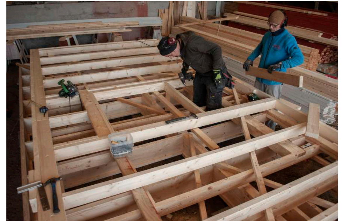
Image 27. Walls were built on top of the floor structure. March 16
