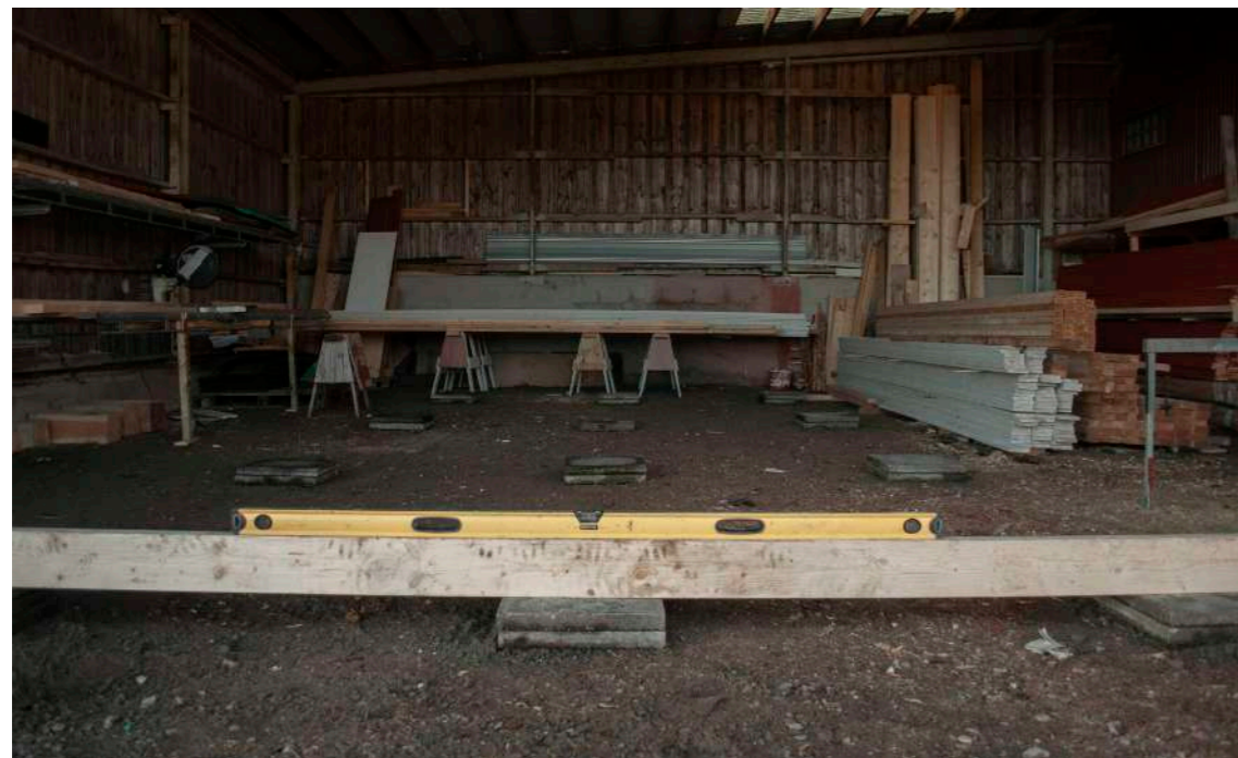
Image 18. The piles were grounded with gravel and sand which eased the process of making each pile perpendicular to the other. March 6
