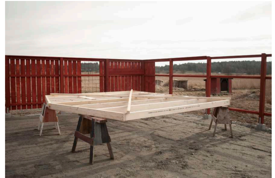
Image 35. Temporary placement of the gables. March 24
