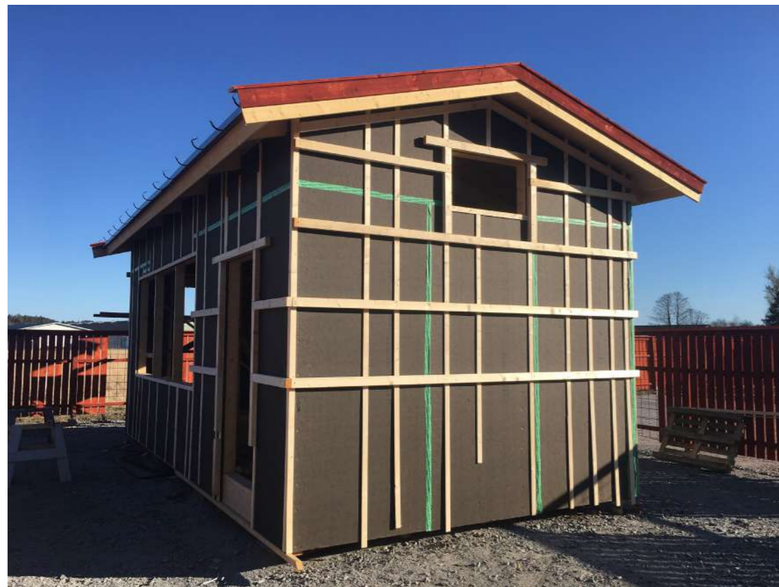
Image 74. Wooden battens mounted on the asphalt. April 22
