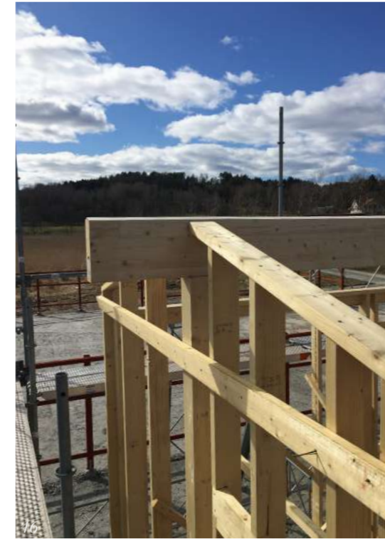
Image 46-47. When the ridge beam was mounted on the two gable walls and the rafters were mounted on the beam, an error was discovered. The two gables were askew, making the rafters too long for the house causing them to fly in the air. March 30
