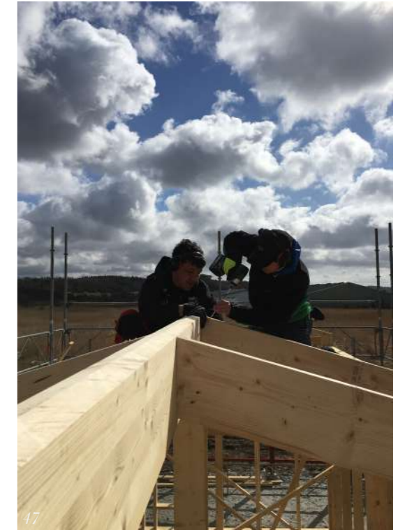
Image 46-47. When the ridge beam was mounted on the two gable walls and the rafters were mounted on the beam, an error was discovered. The two gables were askew, making the rafters too long for the house causing them to fly in the air. March 30
