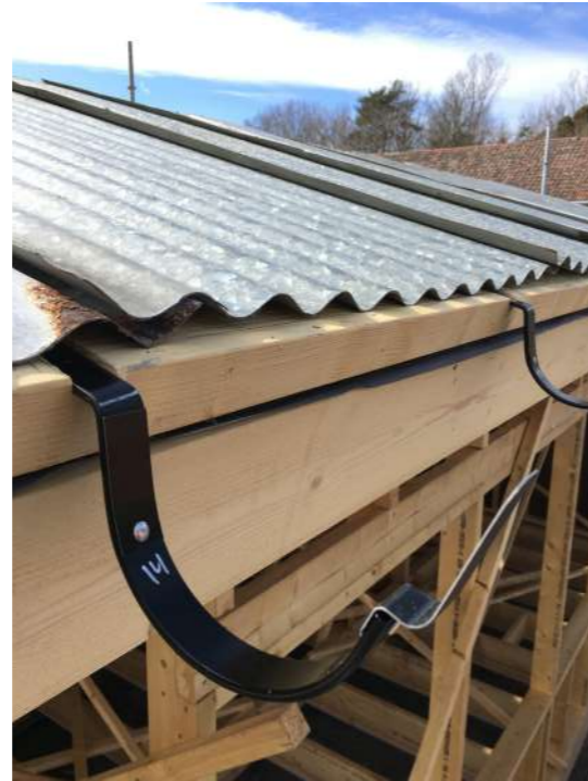
Image 64. Mounting of new gutter brackets. April 14
