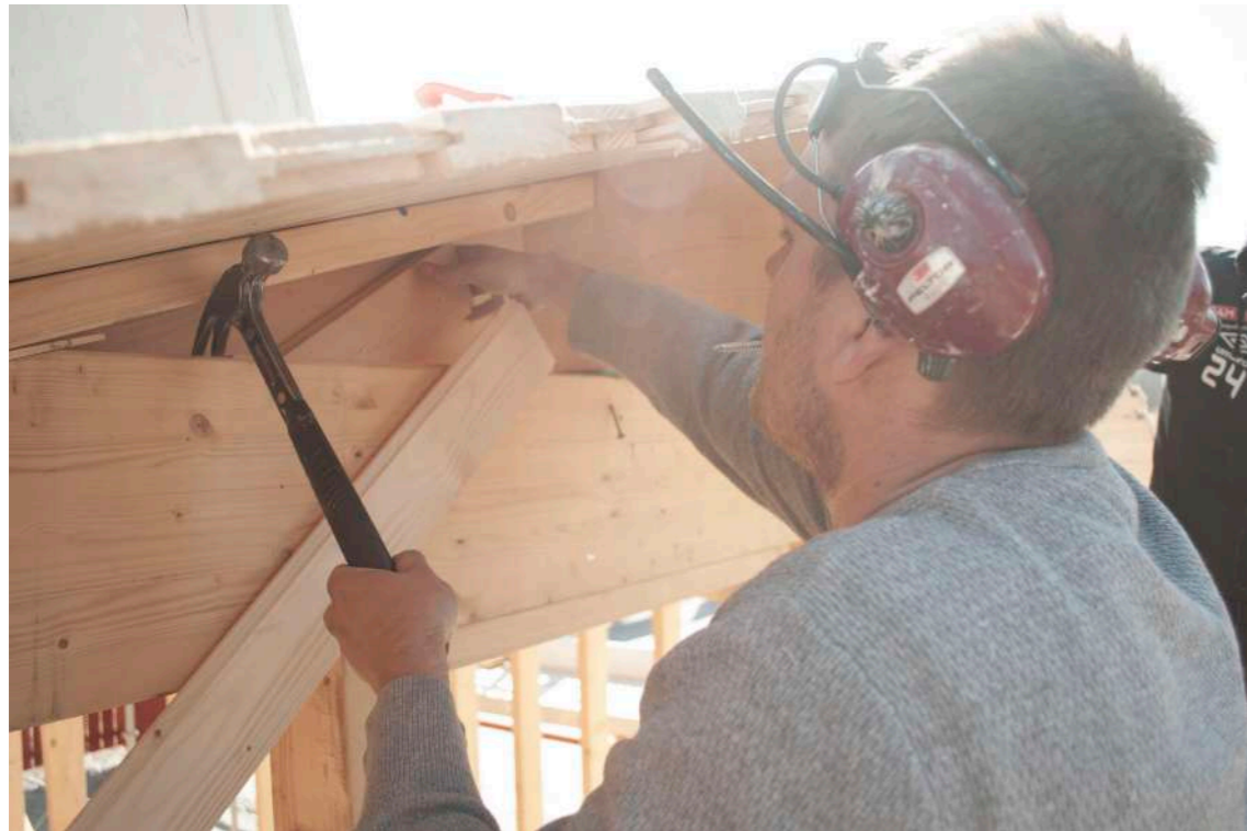
Image 55. Carpenter fixing the flying ridge beam. April 6
