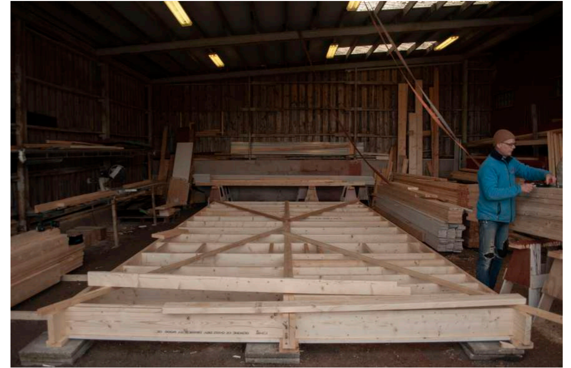
Image 26. Assembled floor structure. March 12
