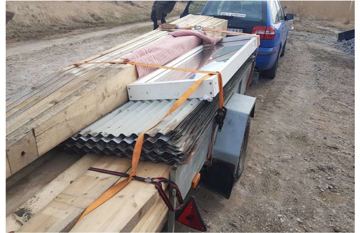
Image 39. Delivery of reused materials. March 24
