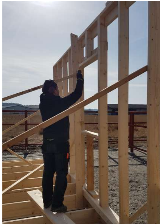
Image 37. Raising the walls. March 25
