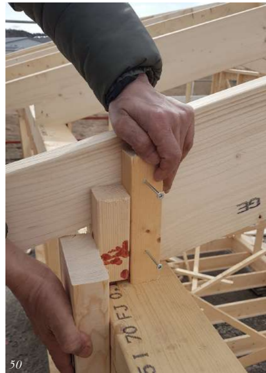
Image 50-51. Some tips and tricks from one of the carpenters. If several similar parts are to be constructed or mounted, it is easier to get it right by creating different templates to use. April 1
