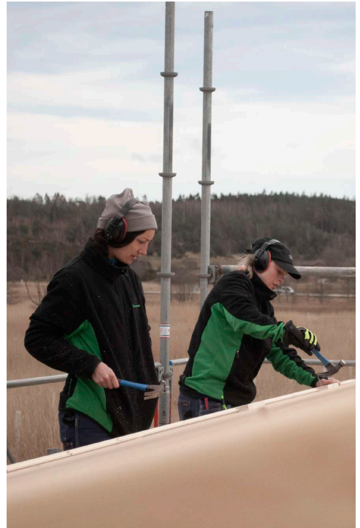
Image 75. Mounting of the tongue and groove. April 1
