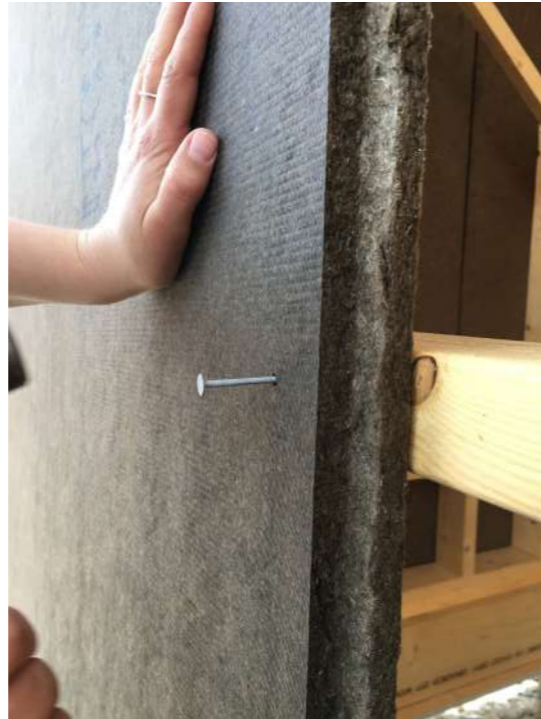
Image 70. Mounting of Asfaboard. April 15
