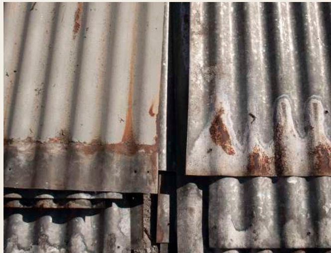
Reused metal sheet roof
