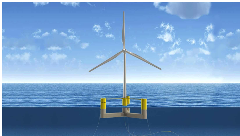
Figure 1.2: The UMaine VoltturnUS-S semi-submersible reference platform supporting the IEA-15-240 wind turbine. Image courtesy of the University of Maine.
