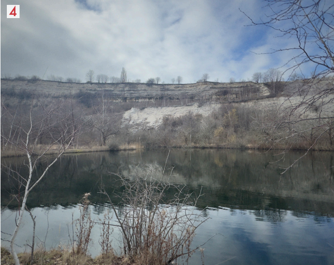
Fig 11: Water retention pond
