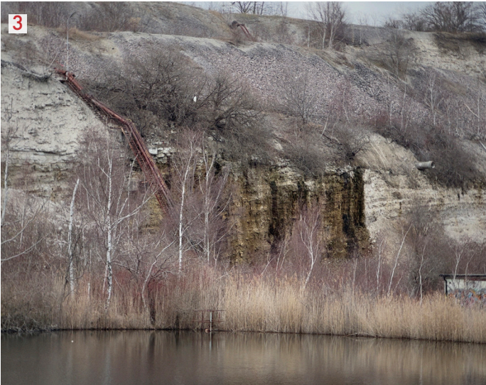
Fig 10 : Water pumb pipe and vegetation along cliff edges
