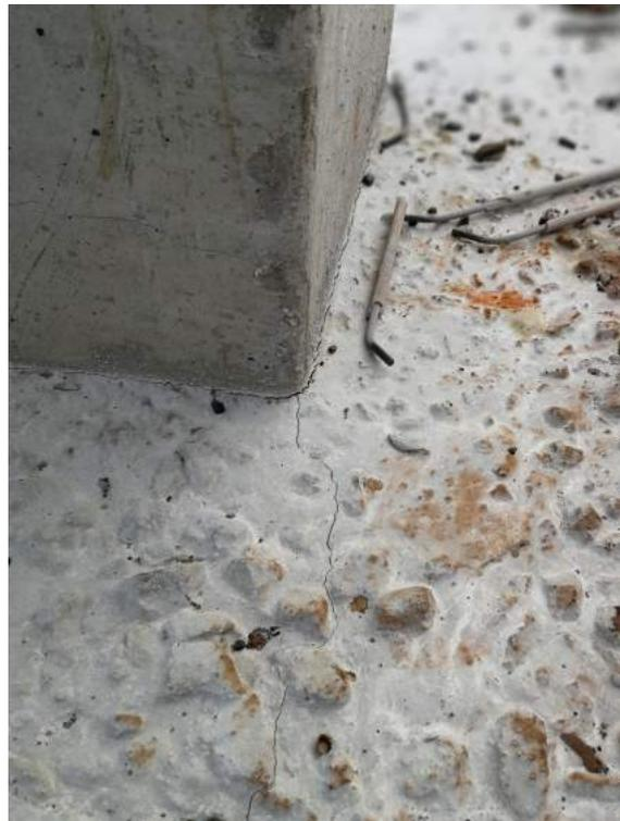
**Figure 6.2:** Cracks in the concrete slab, spreading out from one of the supportive piles
