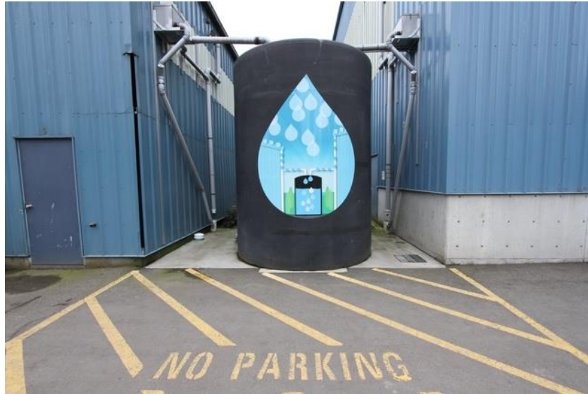
Figur 5. "The Church Point Transfer Station in the Regional District of Nanaimo is Leed gold - this is rainwater collection", foto av Green Energy Futures. Licensierad genom CC BY-NC-SA 2.0 ( https://search.creativecommons.org/photos/268352c0-edd4-4d37-8b48-070723e48e81 )
