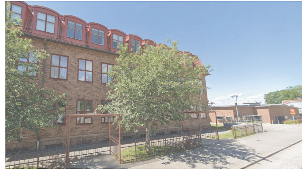
Figure 19: The building housing the music classes for the culture school. Picture retrieved from google streetview.
