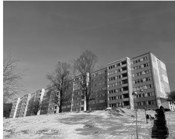
Figure 2: Housing Block at Siriusgatan
