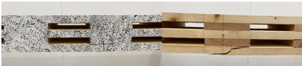
Figure 4-63 Detailed pictures of the failure for Sample 2 of Configuration C. The picture at the left depicts the front side and the right one shows the unpainted backside of the beam.
