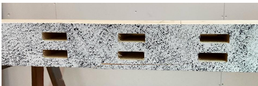
Figure 4-47 Detailed picture of the crack of Sample 2, Configuration B.
