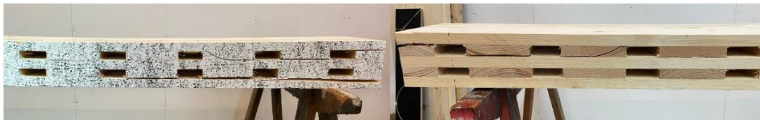
Figure 4-46 Detailed pictures of the failure for Sample 2 of Configuration B. The picture at the left depicts the front side and the right one shows the unpainted backside of the beam.
