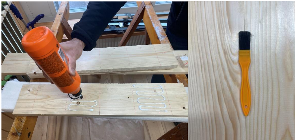
Figure 3-7 Application of the glue on the longitudinal layers at the places where cross-layers will be attached.
