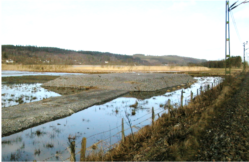
Figure 2.1: Constructed test embankment in Nödinge (Edstam, 2007)
