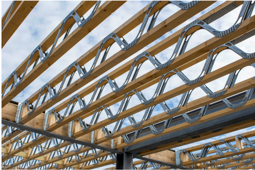
Figure 2.11: Space joist truss (ITW, 2013). Photo © ITW / www.flickr.com/photos/itw-industry
