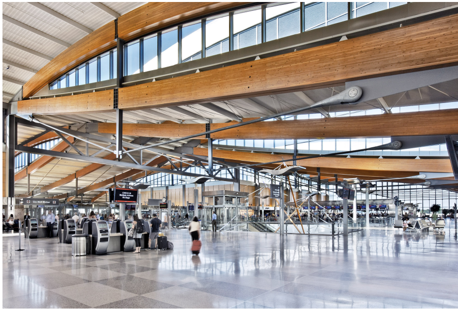
Figure 2.9: V-shaped TSC trusses at the ticketing check in kiosk 02-PD at Raleigh Duram Airport. Photo © Paul Dingman, courtesy of Fentress Architects
