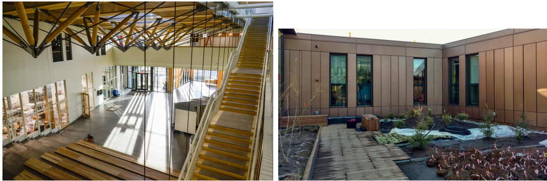
Figure 4.12: Left: The interior atrium with zipper trusses supporting the roof. Right: The roof garden which is supported by the trusses. Photos © Alex Schreyer / UMass
