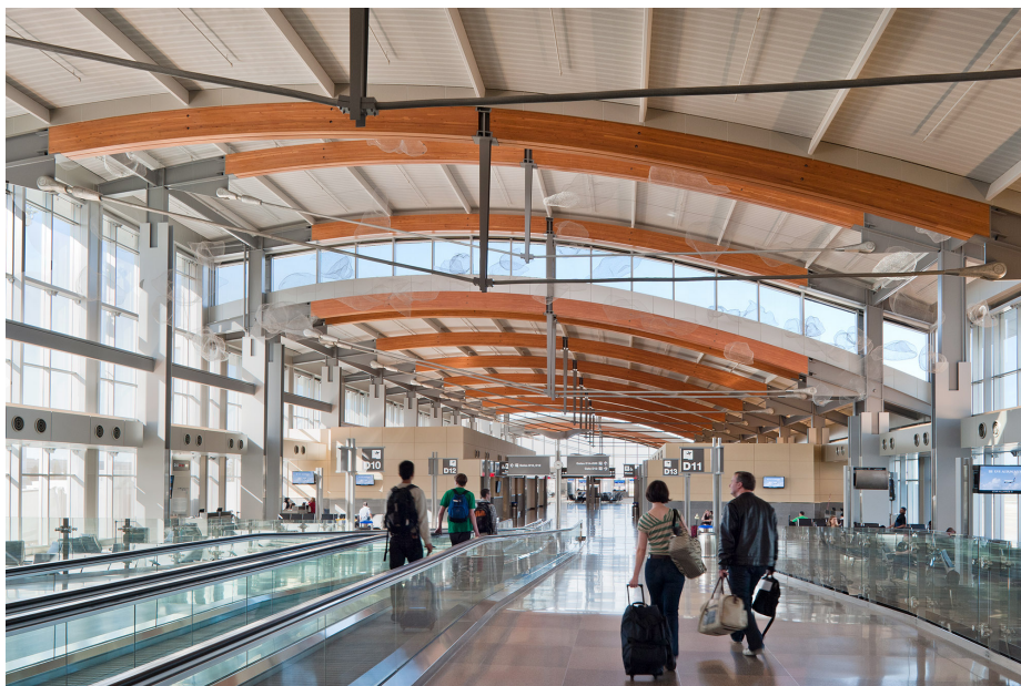
Figure 2.10: V-shaped TSC trusses at one of the concourse at Raleigh Duram Airport. Photo © Brady Lambert, courtesy of Fentress Architects
