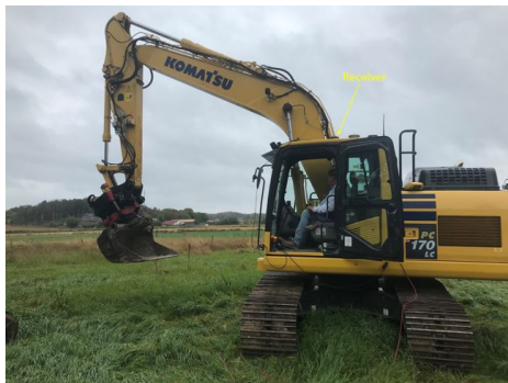
(c) Photo of the excavator showing the placement of the receiver.
