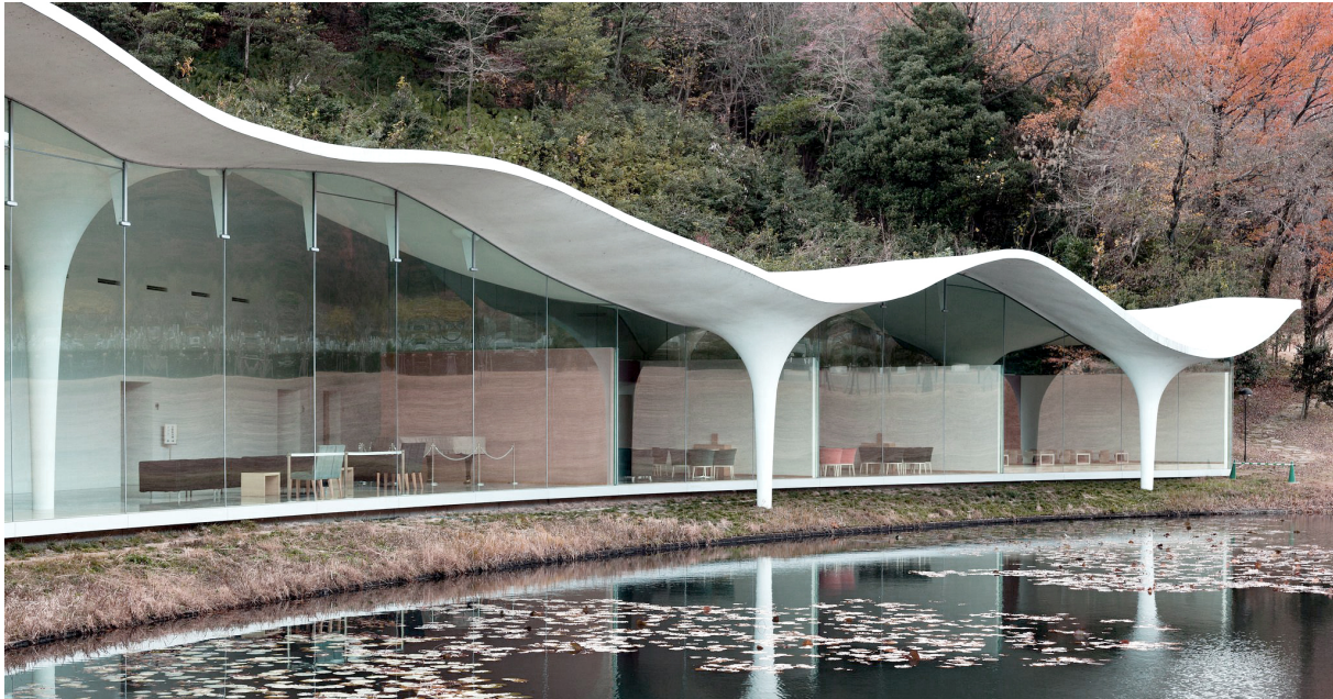
Figure 2.5: Meiso No Mori - Freeform Shell [Toyo Ito/Mutsuro Sasaki] [34]
