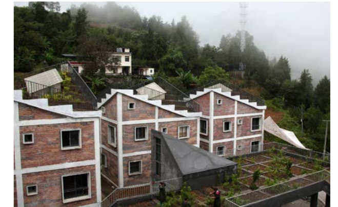
Figure 9. From RUF (2017). Residential houses and garden in Jintai Village [photography]. https://divisare.com/projects/301565-rural-urban-framework-jintai-village-reconstruction
