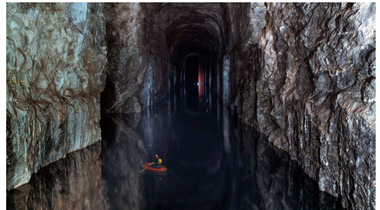
Figure 31. From Göteborg Hamn (2011). Mountain vault for raw oil storage. [photography]. https://www.mynewsdesk.com/se/goteborgs_hamn/pressreleases/historiskt-oegonblick-raaolja-lastas-ut-fraan-goeteborgs-hamn-629841
