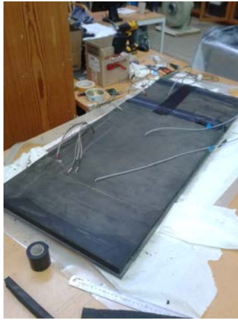
Figure 9.2: Wall after back isolation
