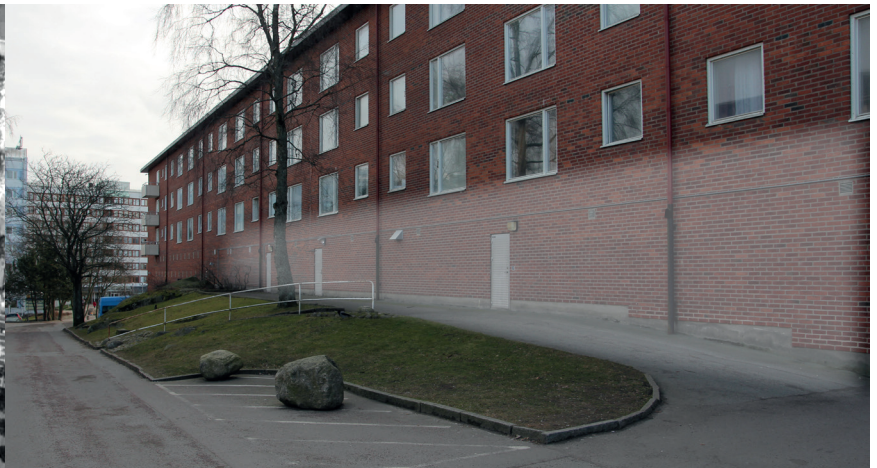
Figure 49. (Author, 2017) Example of facade with potential for public use- north east corner of Block 2
