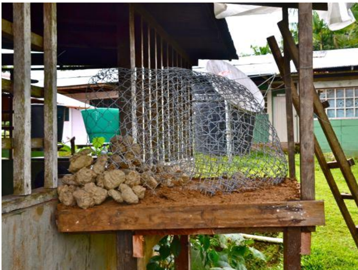
Figure 12: Steel mesh reinforcement
