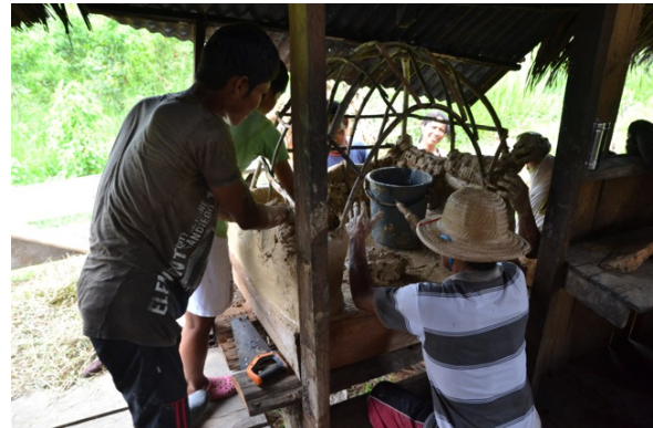
Figure 11: First model with flexible tree branch reinforcement
