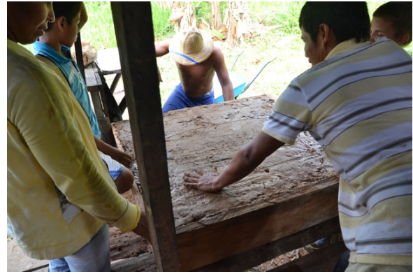
Figure 9: New base for the construction
