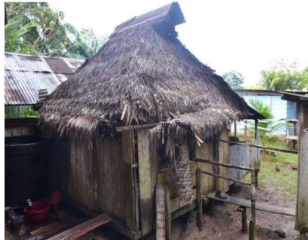
Figure 4: Exterior of a household kitchen in Puerto Rico
