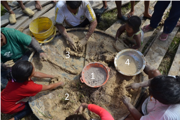
Figure 10: Kneading process with ashes (1), grass (2), clay (3) and water (4)
