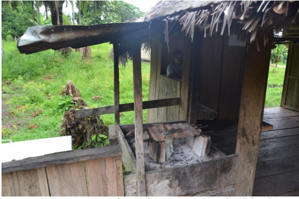
Figure 8: Previous cooking place in minor school kitchen
