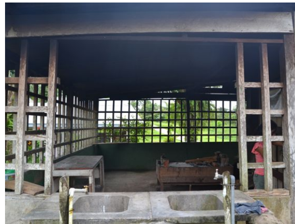
Figure 6: Interior of the major school kitchen
