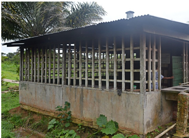
Figure 5: Exterior of the major school kitchen
