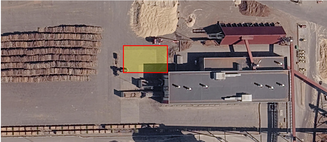
Figure 4.3: New charger area highlighted in yellow.
