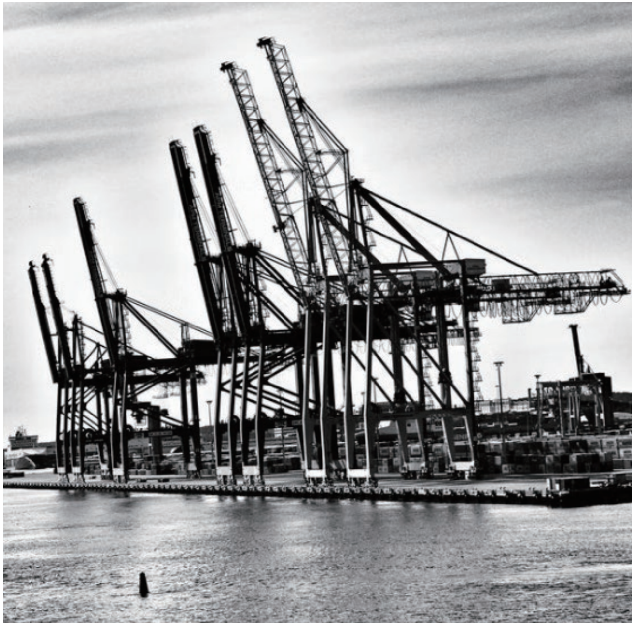
Figure 20: Cranes in Gothenburg Source: FOLKEZINIPHOTO
