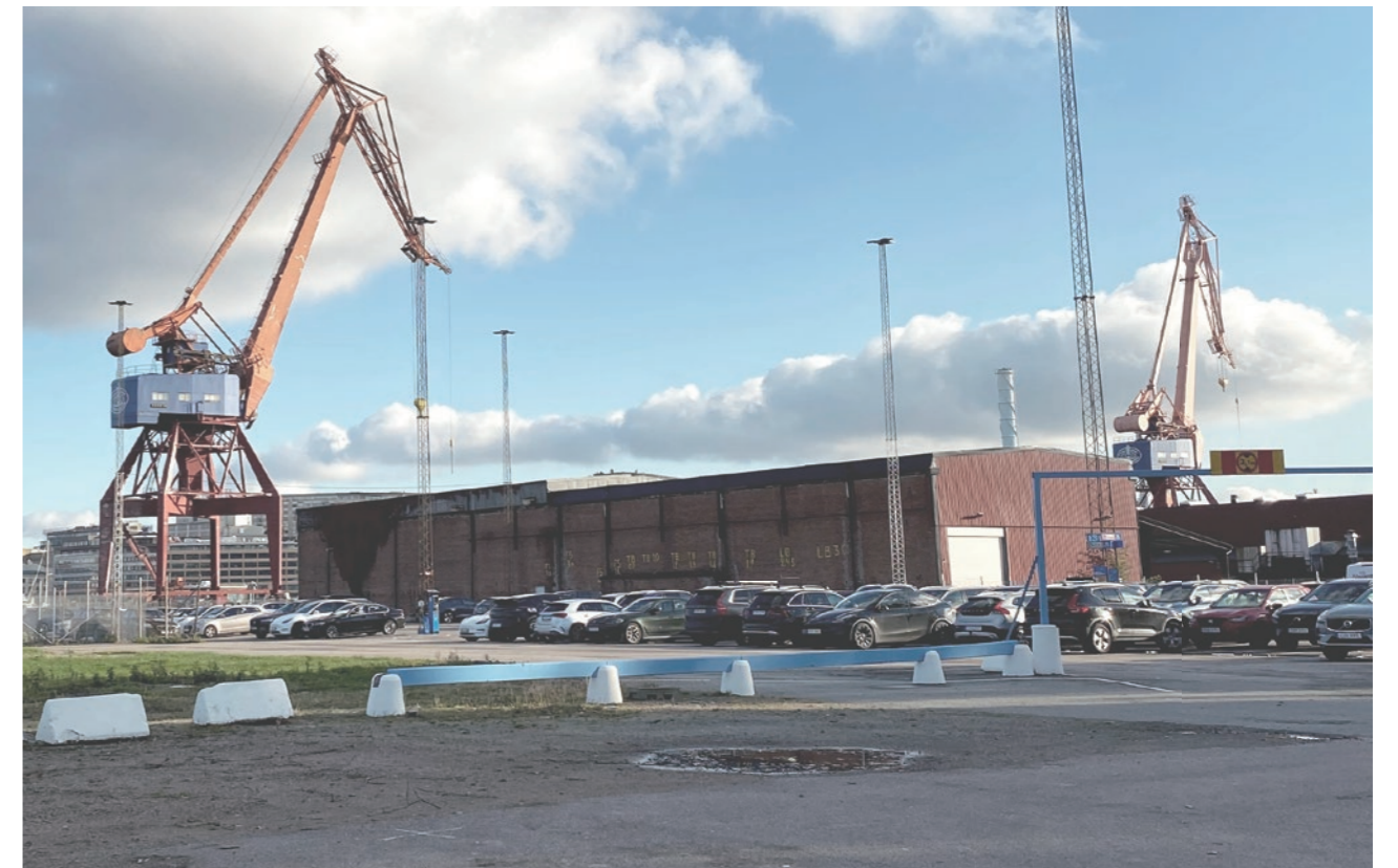
Figure 2: Industrial facilities in Lindholmen
