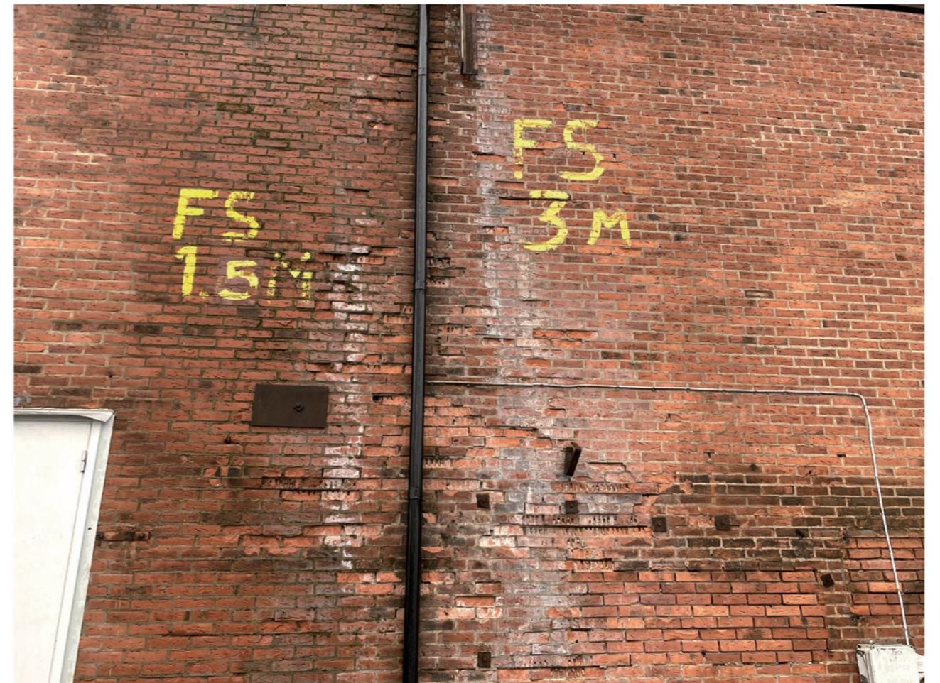
Figure 19: A no-functional factory building
