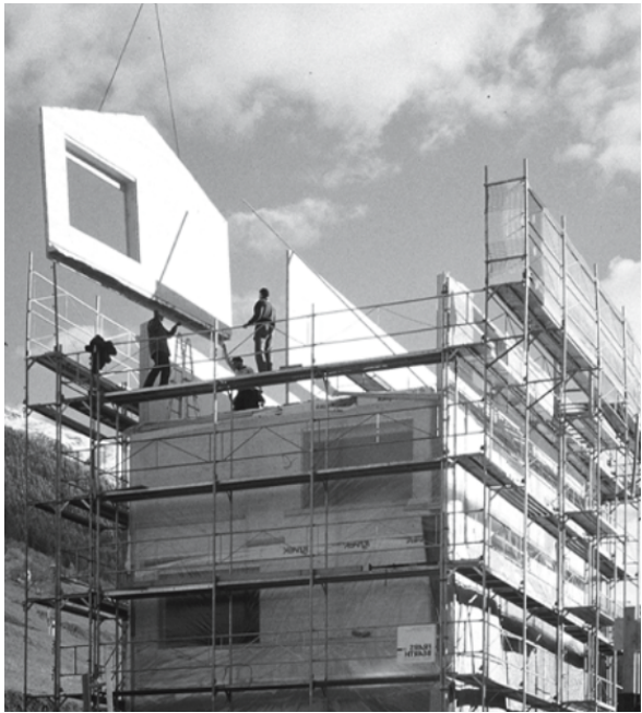
Mounting process and Vertical section Constructing Architecture (Deplazes, 2005)
