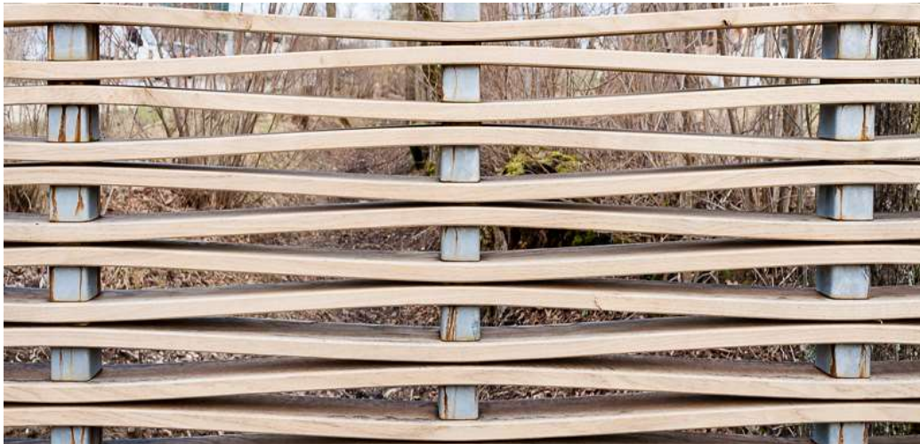
Figure 3.8 Railing structure with distancing (Makiol Wiederkehr, 2014a). Used with permission.
