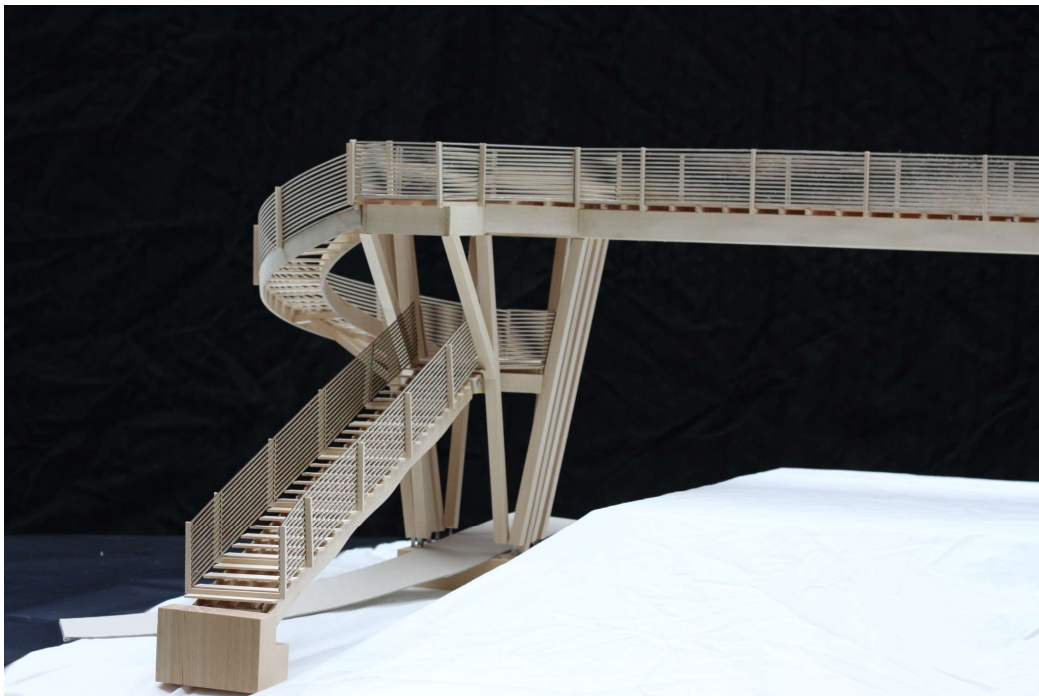
Figure 7.5 Viewing platform and pathway down to the ground level. The straight staircase also contributes to the horizontal stability.
