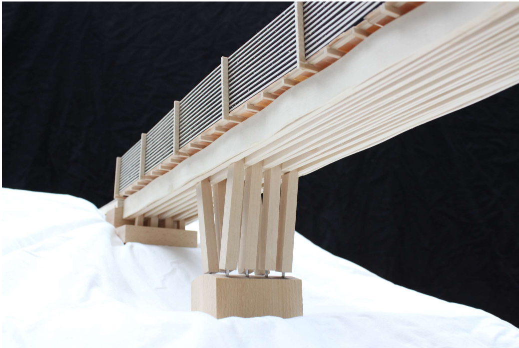
Figure 7.4 The supports are integrated into the superstructure creating a homogeneous appearance.
