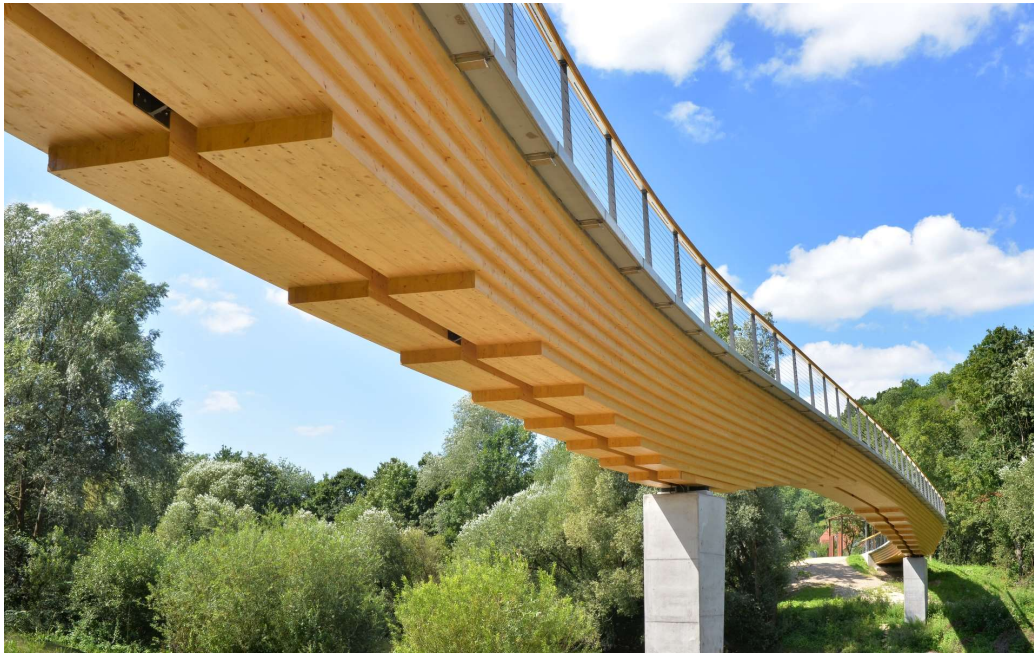
Figure 3.3 Neckartenzlingen Pedestrian Bridge (Burkhard, 2017). Used with permission. © www.hochbau-fotografie.de
