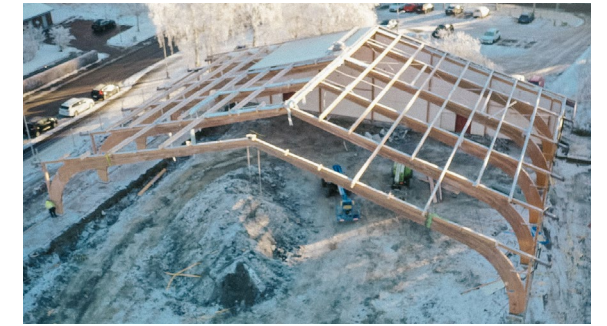
Figure 38. The demolition site (Photo © Niclas Malmeling)
