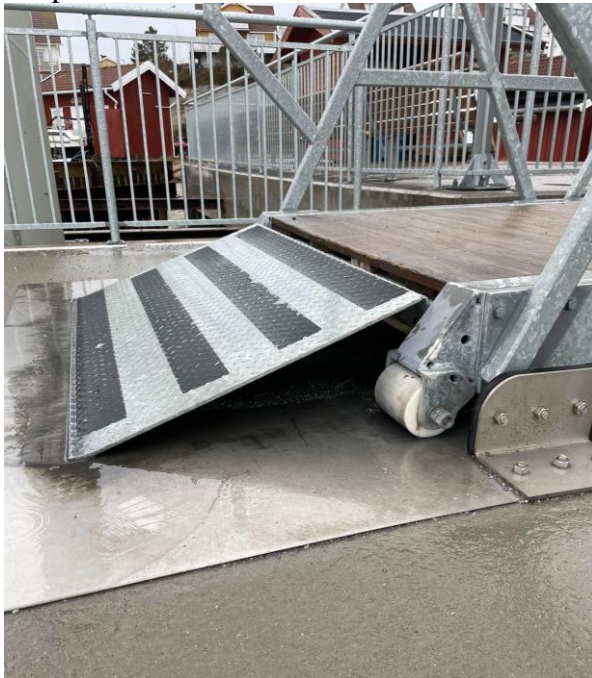
Figure 7 The pontoon and ramp to the pier of the island of Gullholmen (the authors, 2023).
