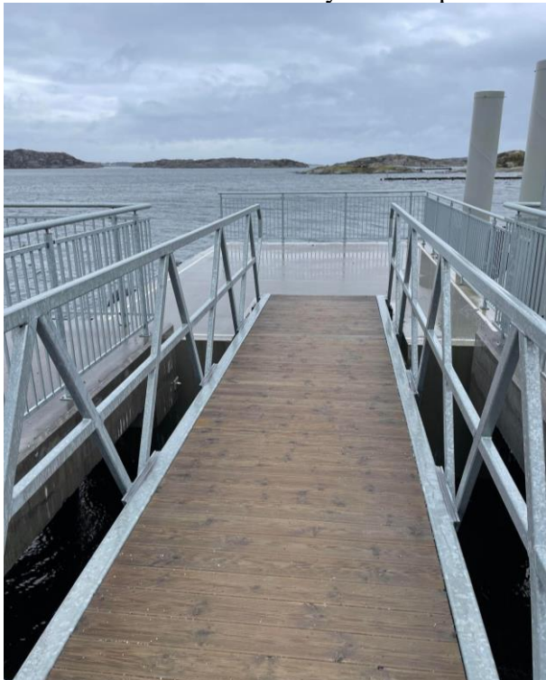
Figure 8 Ramp between the pontoon and the pier of the island of Gullholmen (the authors, 2023).
