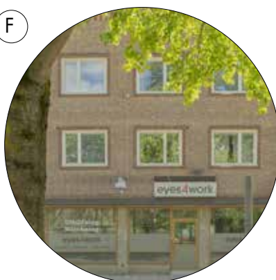
A 12 meter high brick structure.
