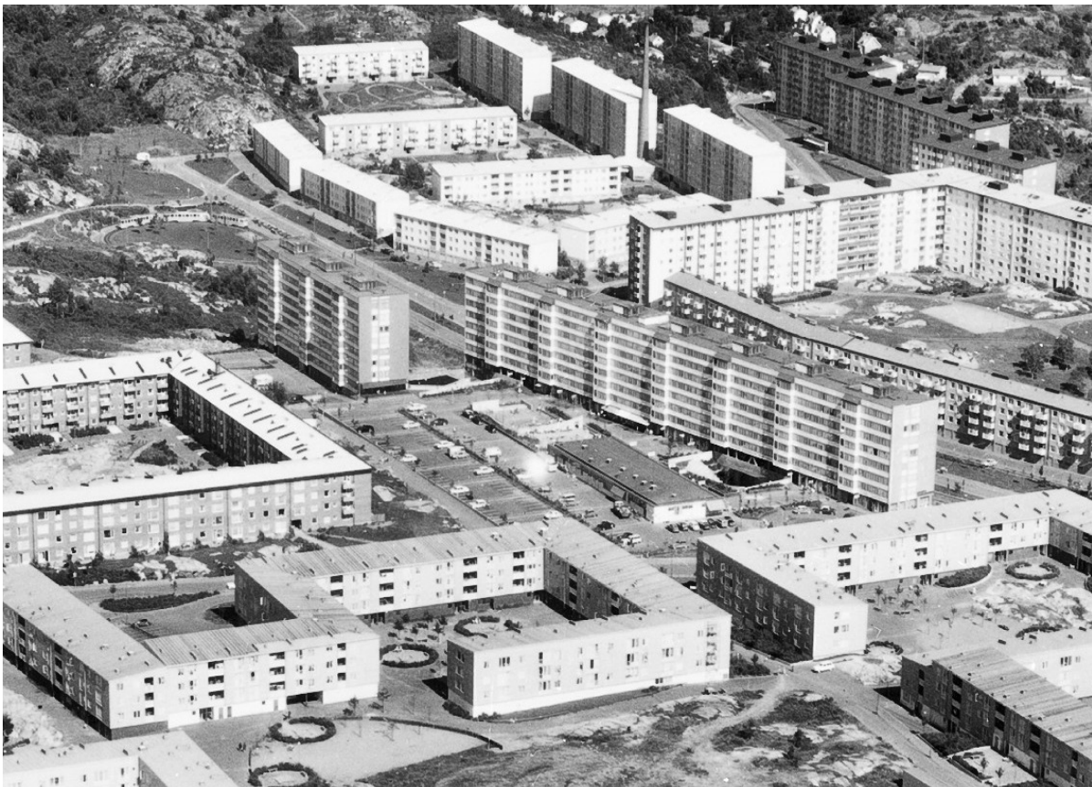
View of Friskvåderstorget during the construction of Norra Biskopsgården. The amphitheater is visible between the grocery store building and the long high rise building (Flygfoto AB)
