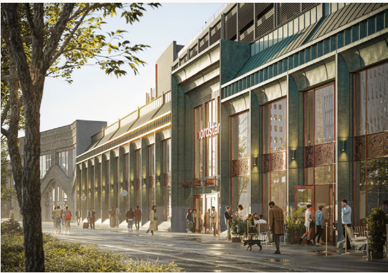
Figure 10 Northern Entrance of Nordstan. (Nordstan, n.d.)
