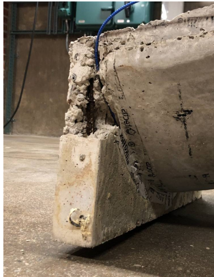
Figure 3.8: Two flaws in the cast prototype element: (i) void in the abutment due to inadequate compaction, (ii) gap between abutment and ground due to a twisting geometry.
