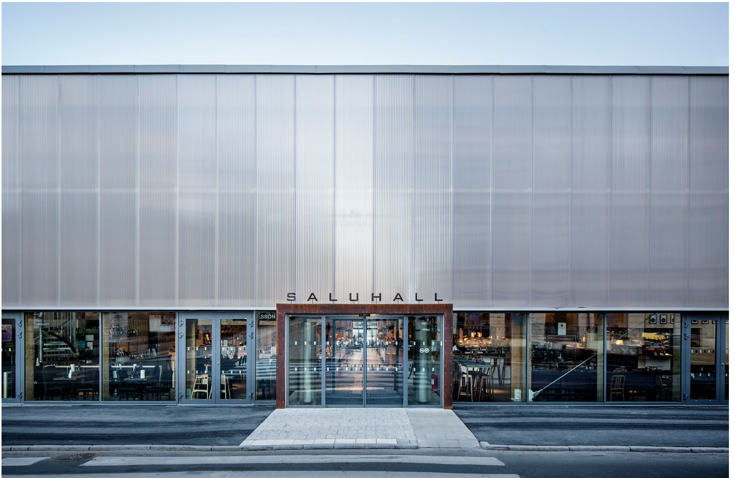
exterior view (Figure 4)
