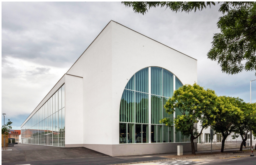
exterior view (Figure 7)
