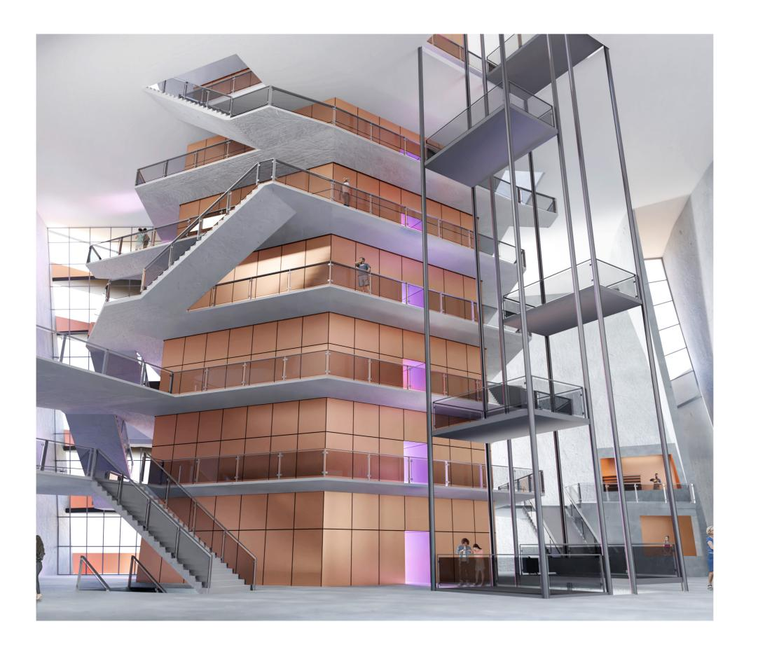
You ascend the building upon the custom platform elevator that transports you to one of the four lobbies. The elevator is basically a periodic path on which platforms travels in one direction slowing down on floor levels for you to get on or off. The lobbies feature a terraced stair situation letting one continue the journey upward through the rooms or enter ones seat in the auditorium. All lobbies have a cloakroom, café, bathrooms and every level has an balcony looking towards the Thames.
