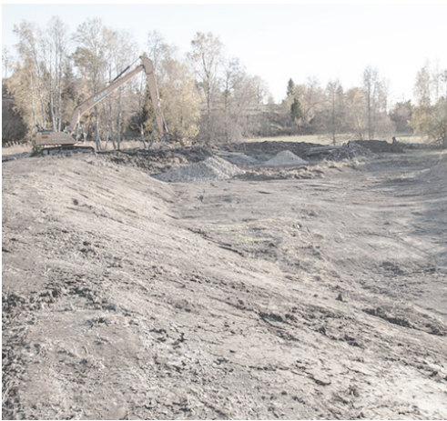
Newly constructed soil Embankment (Söderman, 2018)
