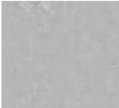
Concrete ground in atrium
