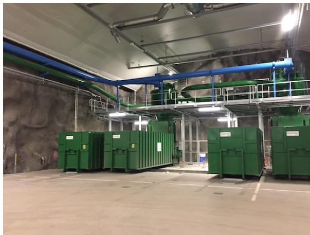
Figure 3.9: Inside of the terminal of Plant 1. The blue pipes carry air and the green carry waste.
