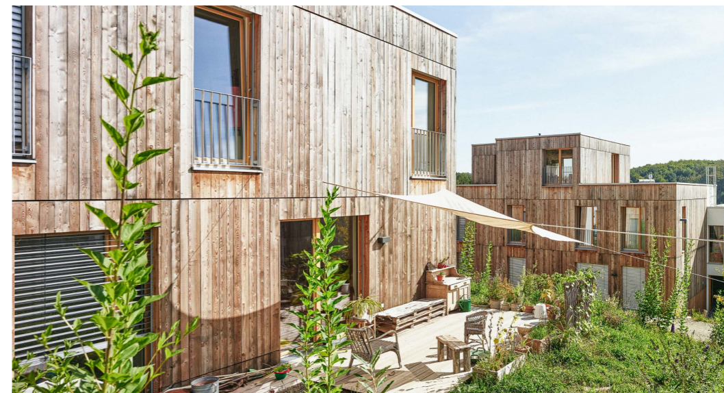
Fig. 20. Closeup photo of the larch wood cladding and a private patio, embedded by greenery. Photo by Kurt Hörbst (2018a).
