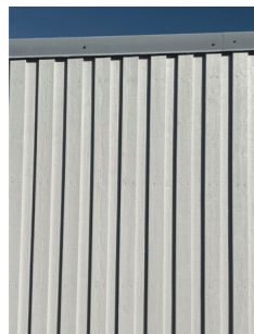
Timber cladding On the sides and back of the garages
