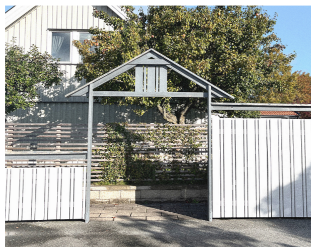
Fig. 63. Existing portal and plank between the parking lot and a pedestrian path.
