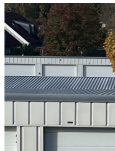
Corrugated metal roofing sheets Total area: ca 2770 m 2
