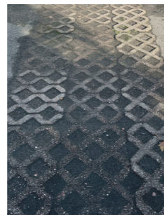
Permeable paving Ca 40-80 m 2 per parking lot
