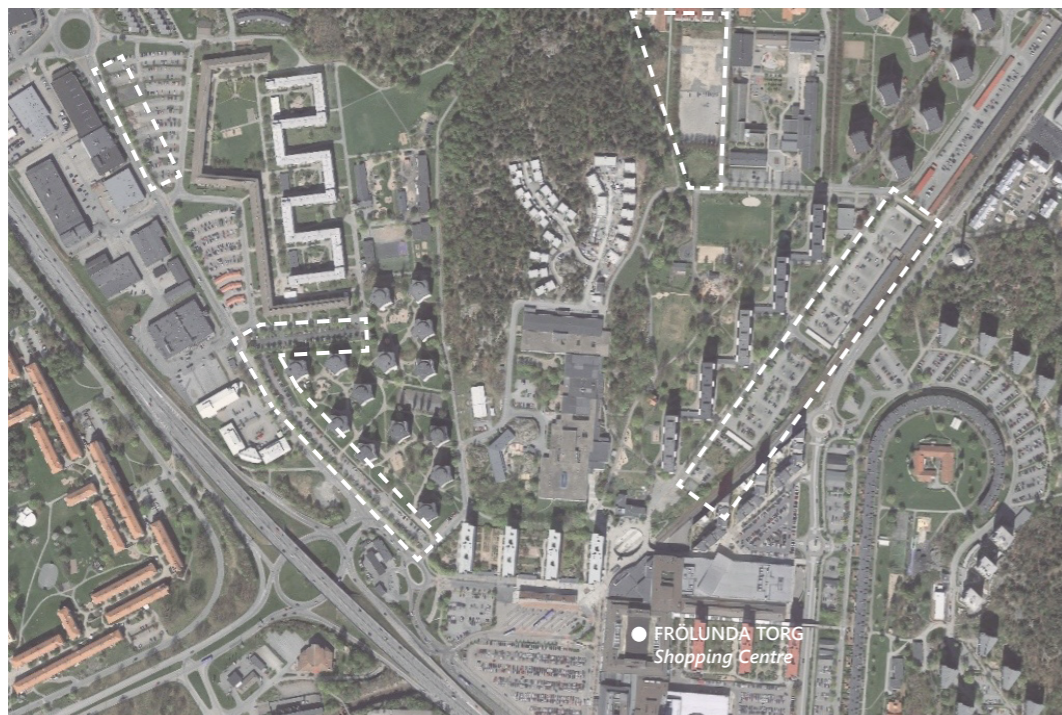
Fig. 8. Aerial view of Frölunda Torg in 2014 (Google Earth Pro, 2014).
