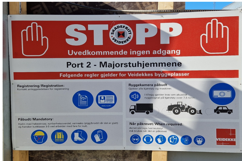
Figure 4.6. Safety requirements are displayed at one of the gates to the construction site. Rearview cameras and audio signals are required for all vehicles that reside within the boundaries of the construction site (middle right of the sign). Own photograph.
