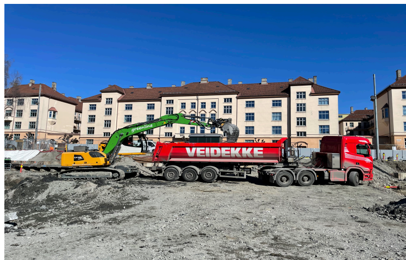
Figure 4.3. The cable crawler excavator loading a truck. Own photograph.
