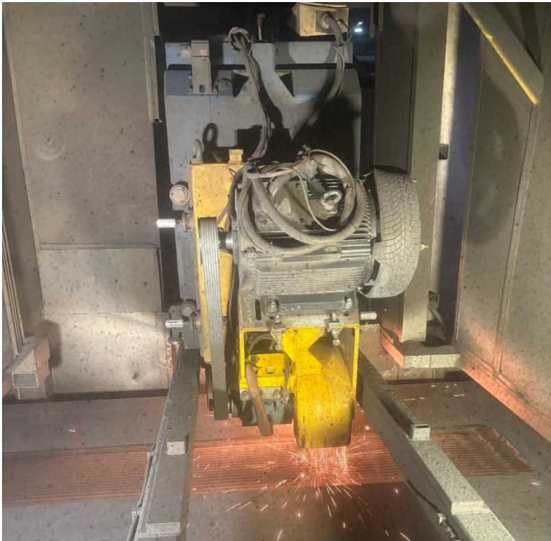
Figure 18: 90° grinding in process
