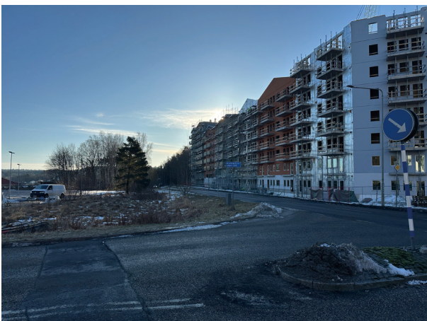
05 The building next to the site
