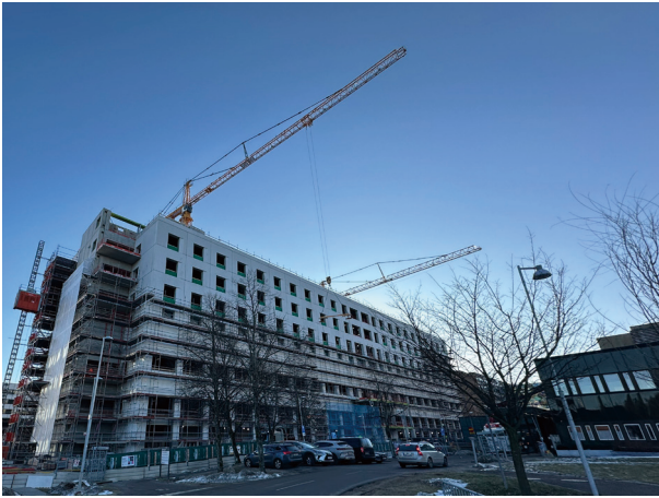
01 the Hospital under Construction
