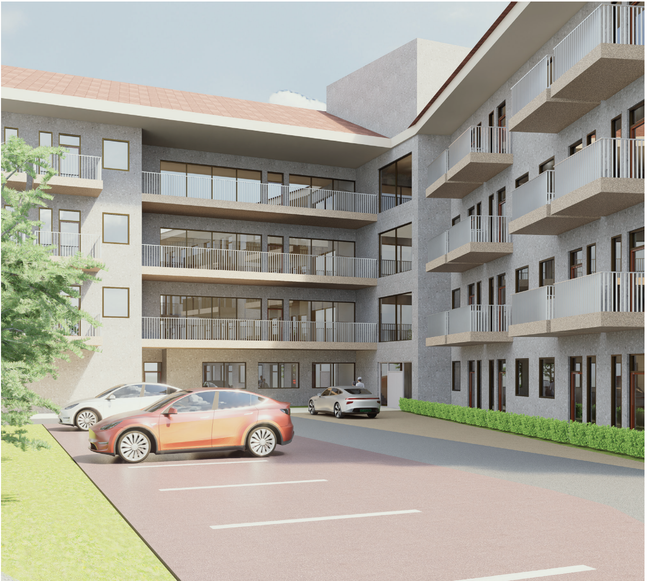
The path to the main entry - for the parking delivery
