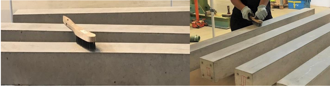
Figure 7.6 Surface preparation of beams for FRP strengthening.
