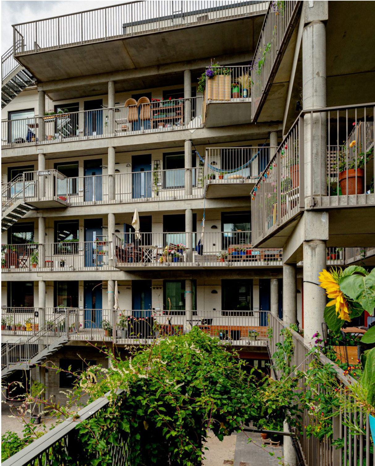
Figure 8. [Sofielunds Kollektivhus] (Lukac, n.d.) The facade towards the yard with access balconies and shared outdoor space
