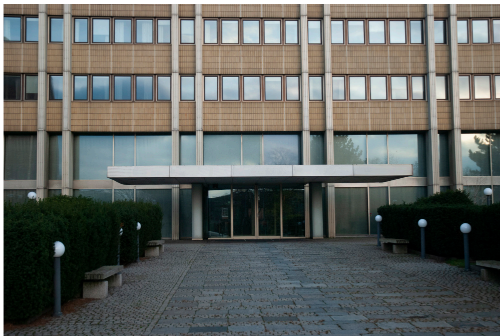
FIGURE 25 SKF, old office building from the 60's.
