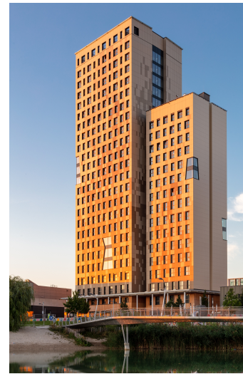
(b) Completed building. [Photograph] by DERFRITZ, 2020.
