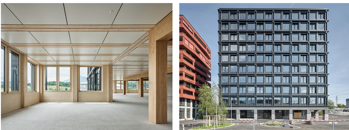
(a) Photo showing structural elements such as columns, beams and TCC slab. (b) Completed building.
