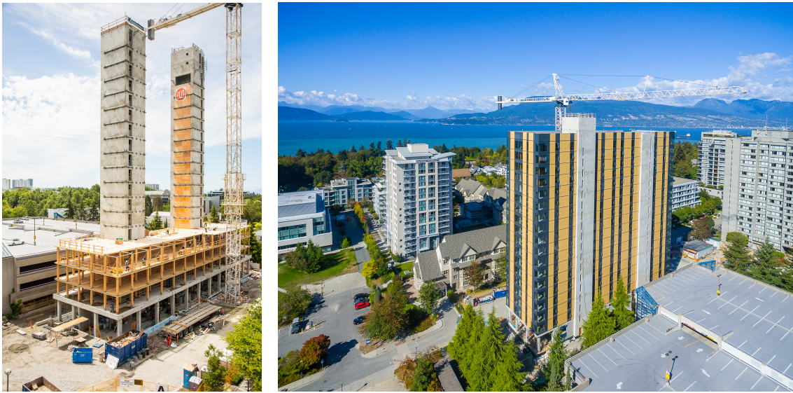
(a) Construction process. (b) Completed building.
