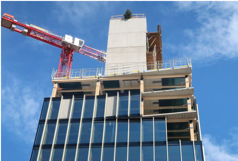
(a) Construction process. [Photograph] by Robert Jockwer, 2018.
