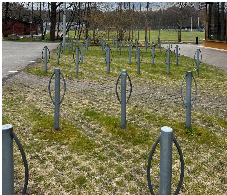
Figure 4: Grasscrete pavers at bicycle parking lot next to Johanneberg Science Park (Picture by authors).
