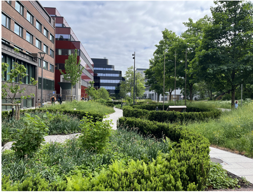
Figure 2: Rain garden complex outside Chalmers University of Technology (Picture by authors).
