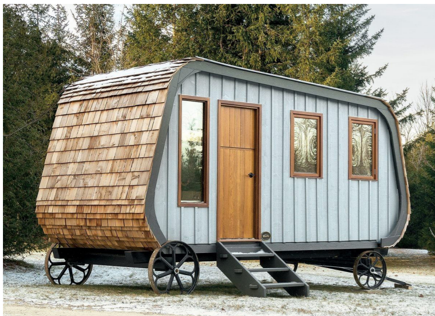
Figure 34: "Shepherd's hut" by Canadian tiny house company Güte is an inspiring example of how to work with the roof bending from front to back, without the house looking like a camper van. The use of wood and detailing associated with old-style huts make it look both modern and traditional. The interior has basic functions beautifully balanced within the minimal space.
