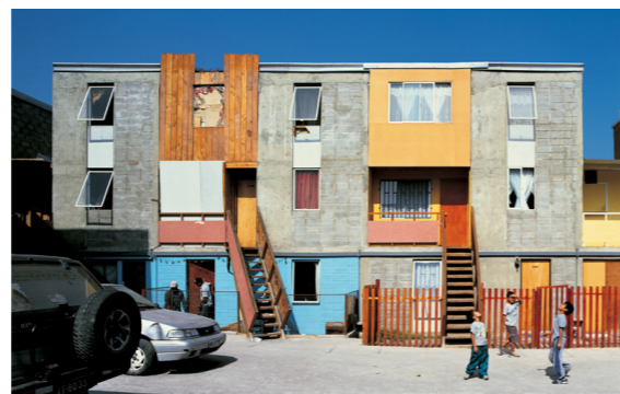
Figure 13: The project Quinta Monroy (2004) by studio Elemental makes use of the building-capacity of the inhabitants to be able to offer housing for half the price (Lundquist, 2017). The row houses, located in Chile, originally only contained basic functions such as toilets, kitchen and stairs. Half of the houses were then built by the inhabitants themselves, resulting in a much lower prize as well as in unique designs.
