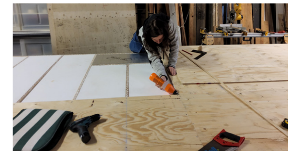
Figure 41: Styrofoam insulation in between studs of 21 mm plywood, and 12 mm plywood for floor.
