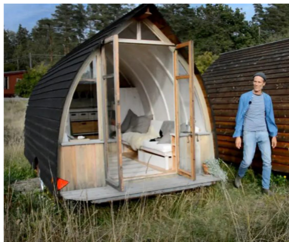
Figure 33: "Kotten" ("The pine cone") is designed by Torsten Grind. It utilises the strength of bent plywood to minimise the weight of the roof. Originally built to function as a summer house by the designer, the little hut has received a lot of attention, why several courses have been held in which participants got to build their own "Kotte". A "Kotte" can be built in 13 days by 3 people, why it serves as an inspiration for more effective ways of construction.
