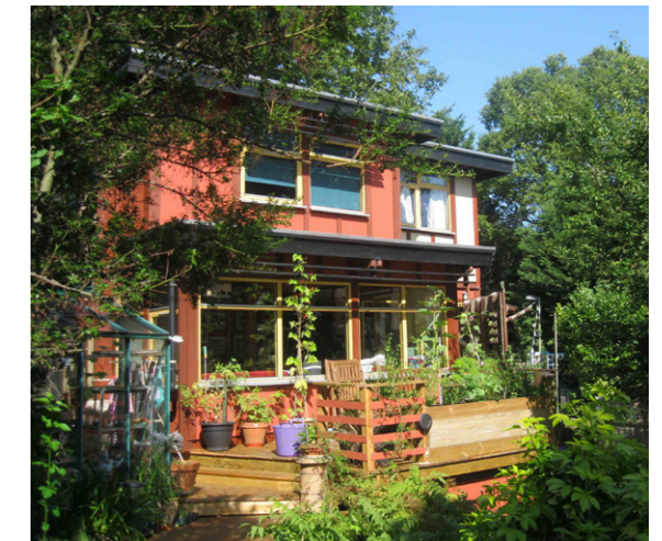
Figure 11: Another example of organized self-building is Walters Way in London, with 13 self-built houses, finished 1986 (Lundquist, 2017). The architect Walter Segal developed a system of construction suitable for self-builders in that it was low-cost, flexible and easy to build. He released a pattern book and list of structural components determined by availability, afford-ability and minimum waste. About 200 buildings were built according to Segal's principles (Lundquist, 2017).
