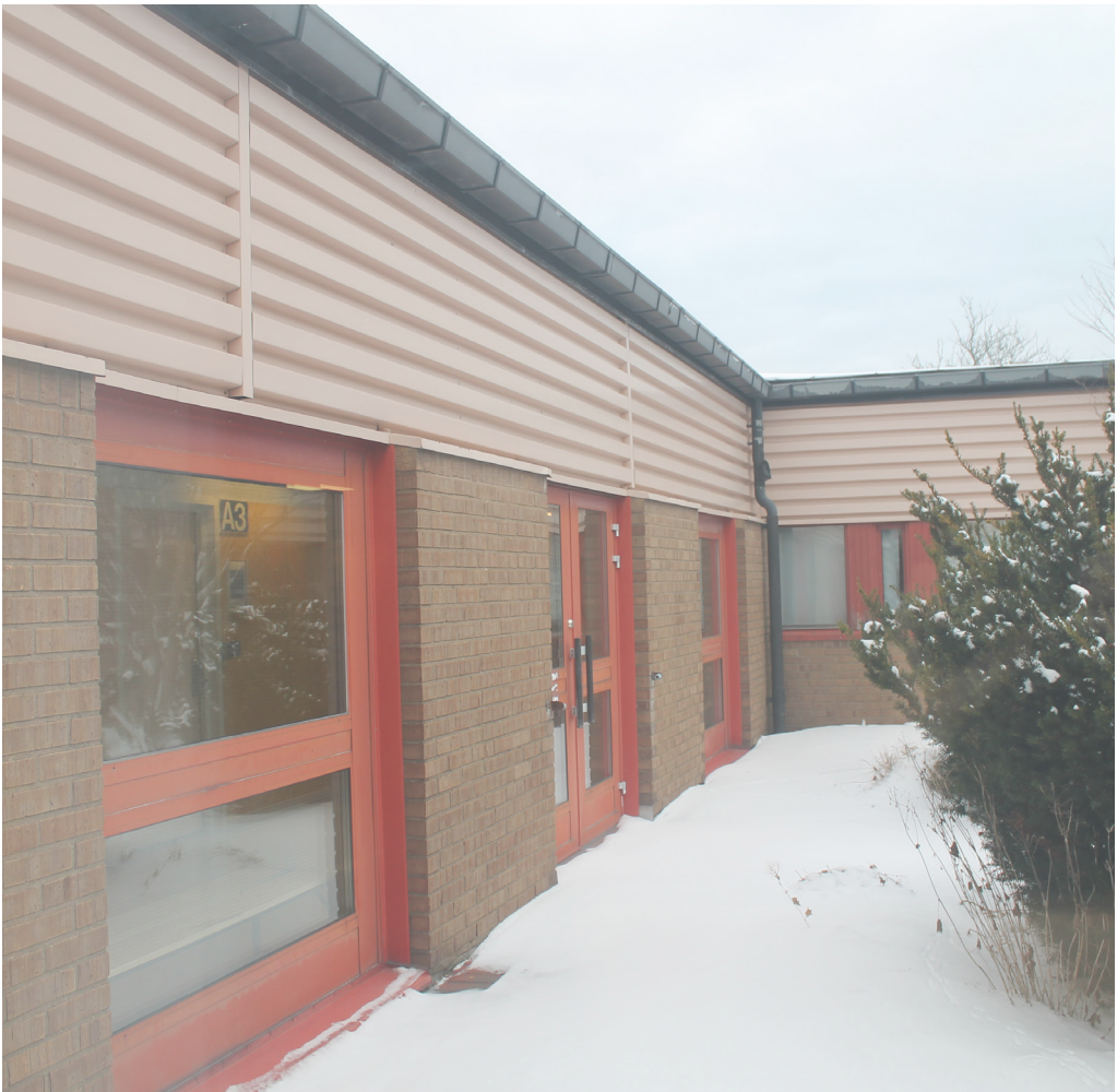
View from the inside courtyard of building 21
