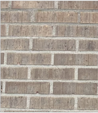
Material: Brick Category: 02. Envelope Reuse Potential: Challenging
