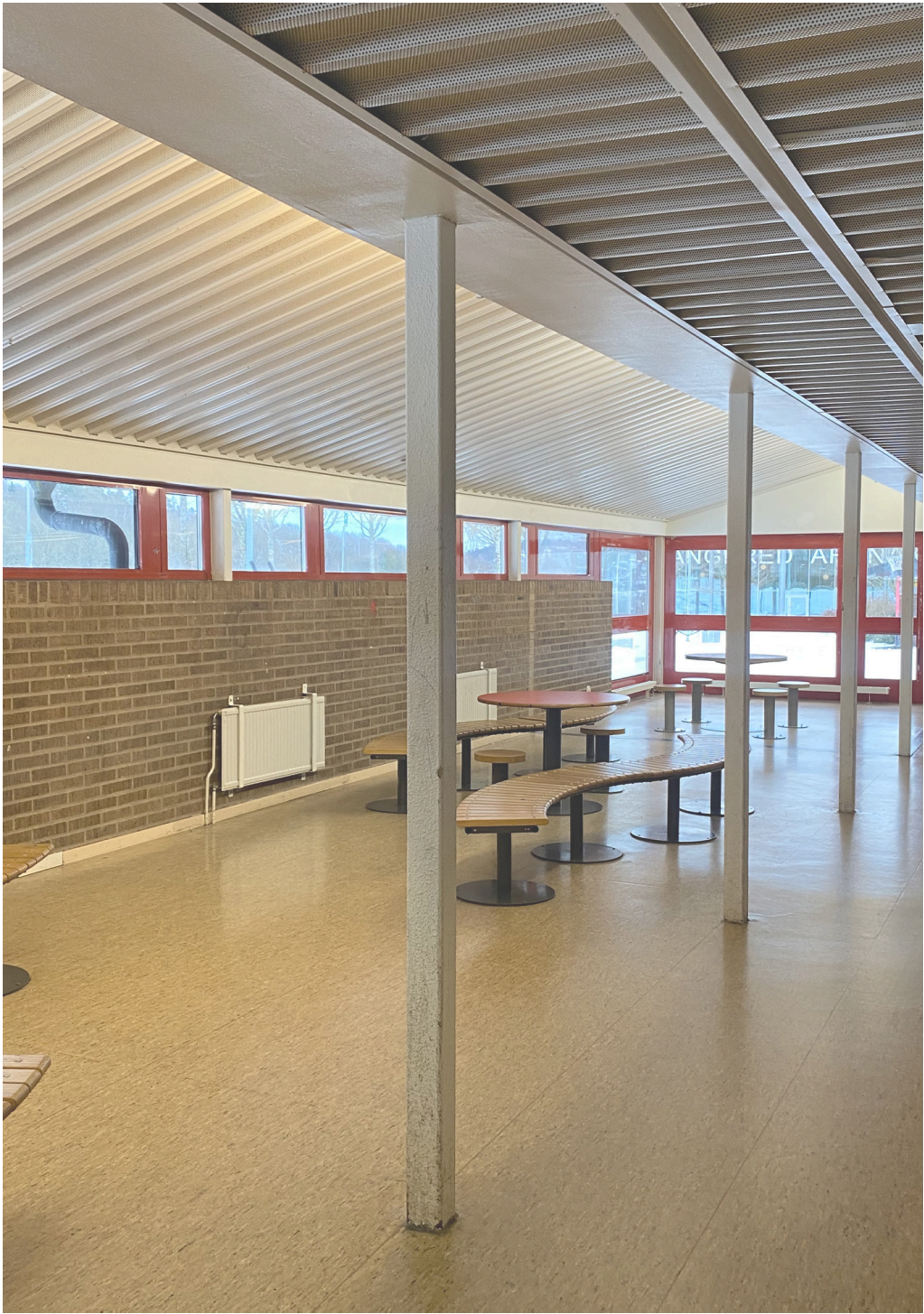
Interior View of Building 21
