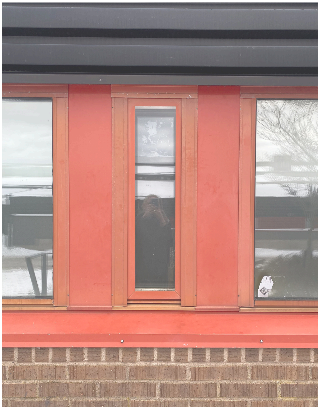
Exterior view of building 21
