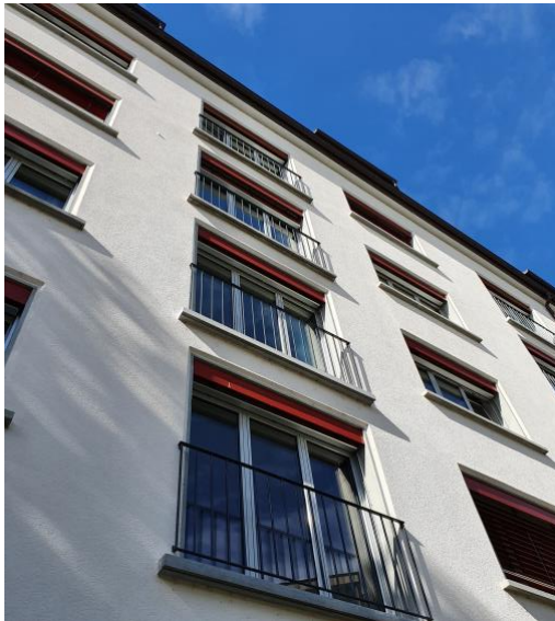
Figure 2.1 Building in Zurich, Switzerland, covered externally by an aerogel-based plaster system. Picture taken by Ali Naman Karim (2019).
