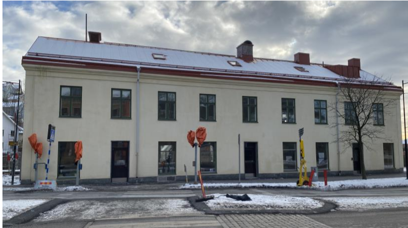
Figure 6.2 The appointed building in February 2021, picture taken during a study visit.
